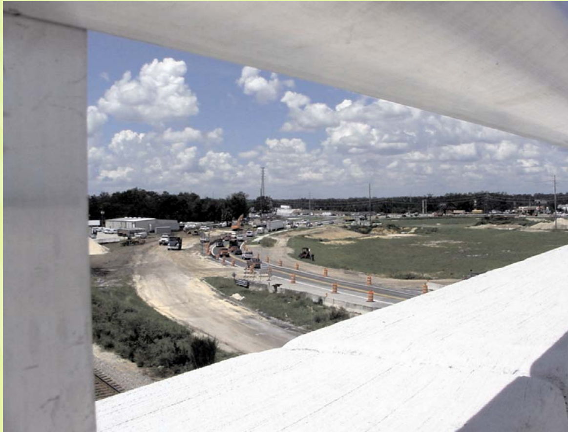
Construction of SR 60 in Bartow - Tim Hunter
