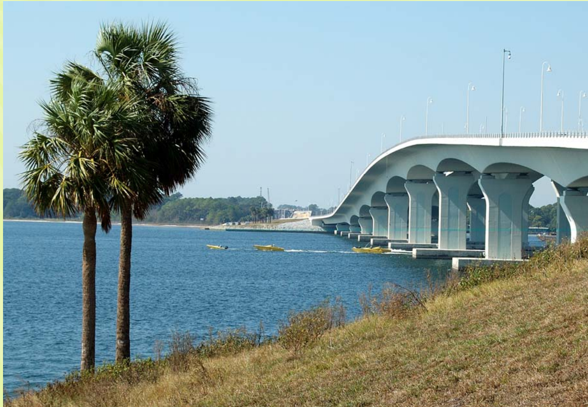
Hathaway Bridge, Panama City - Carole Robertson
